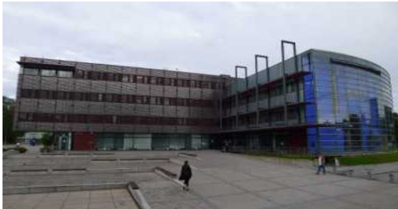
Helsinki University Viikki Campus Library 전경
