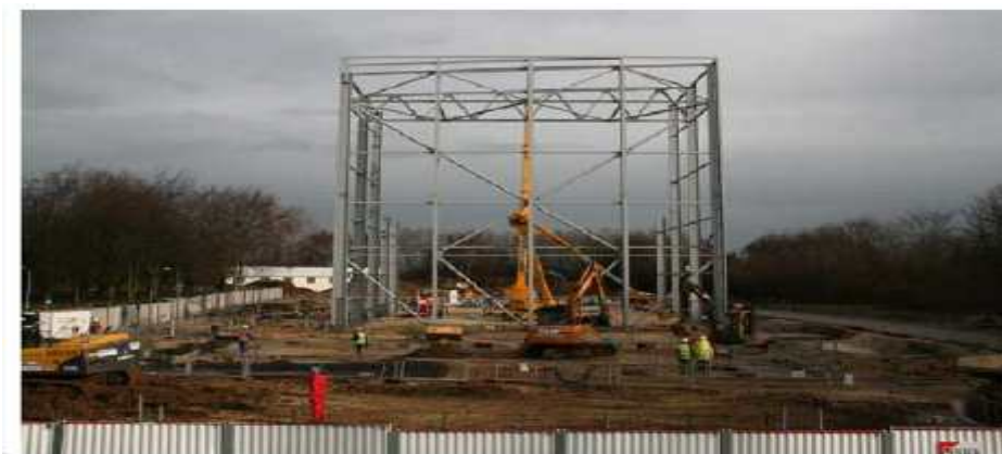
The new newspaper storage building takes shape at Boston Spa
