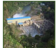
Angat Hydroelectric Power Plant - Auxiliary 4 & 5
