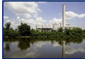
Quezon City Waste-to-Energy
