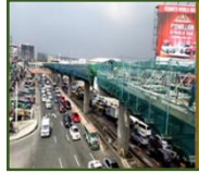
NAIA Expressway Phase (II)
