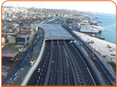
Eurasia Tunnel: Sub-sea link connecting Istanbul continents.
